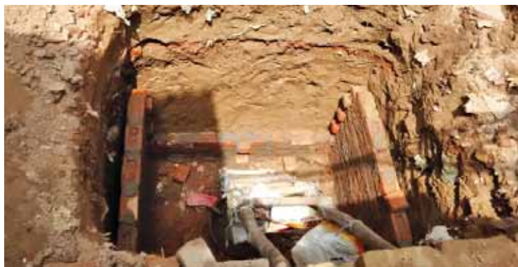
Left: Image showing the constructed toilet at the roof of a house in J.J Colony, Sector-8, Noida, Right: Image of a septic tank getting constructed in one of the slums of Noida.
